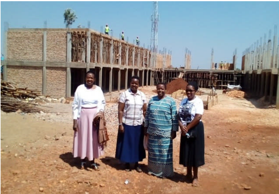
The regional team of Africa visiting the construction of the primary school.
